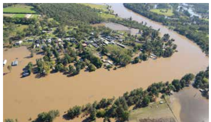
Submerged properties at Gronos Point, March 2021 flood. Source: Adam Hollingworth
