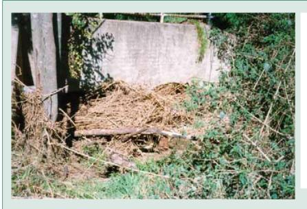
Extensive culvert blocking during the August 1998 Wollongong floods resulted in flood levels with a recurrence interval of greater than a 200 year event being reached despite the rainfall event which caused the floods being equivalent to a 100 year event.
