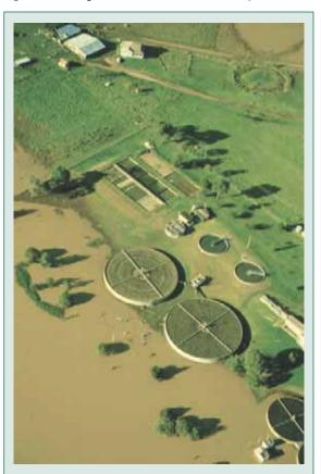
For operational reasons, Sewage Treatment Plants are usually located on low-lying ground. Operational disruption, potential for pollution or damage to critical components due to frequent flooding may be limited in some circumstances by containment within a levee (providing there is no effect on others in the floodplain by building the levee).
