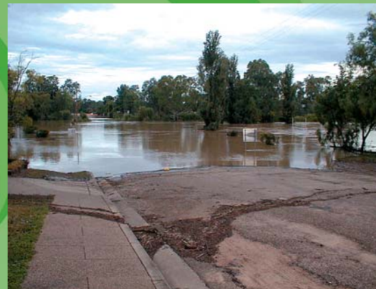
Transport disruption from flooding
