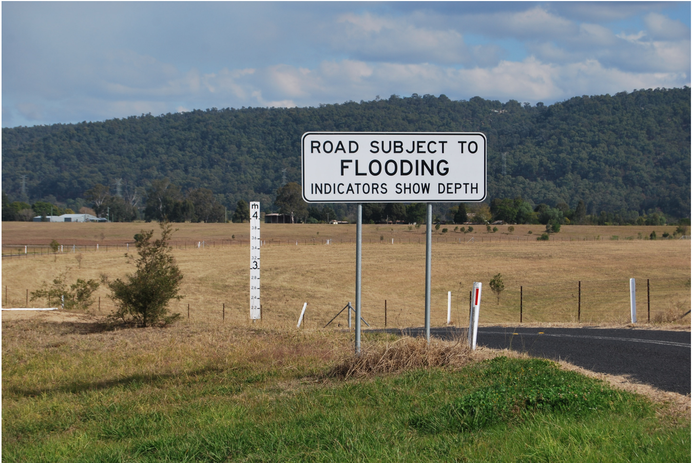
Flood sign and depth indicator in the Penrith / Emu Plains floodplain of the Hawkesbury-Nepean Valley showing inundation levels. Image: Western Sydney University 2019
