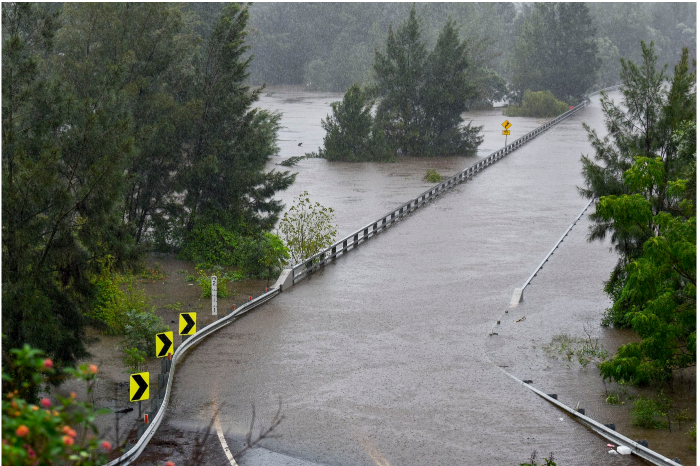
Yarramundi Bridge under floodwater, 10 February 2020. Image: Adam Hollingworth
