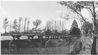
Gosling Creek Dam
