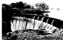
Spring Creek Dam
