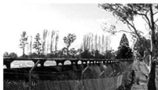
Gosling Creek Dam
