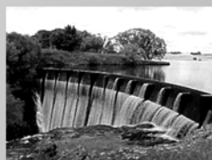
Spring Creek Dam
